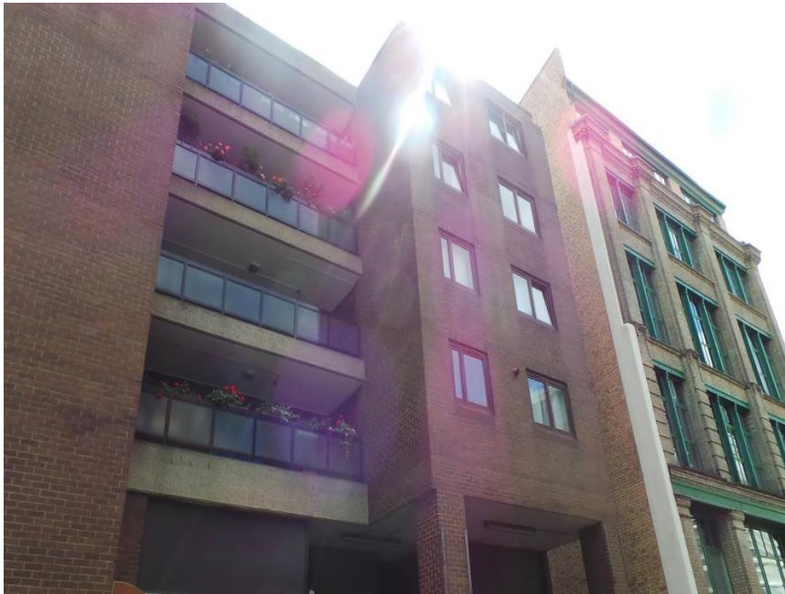
Figure 1; Windows 126 -128, 130, 132 and 134 at 10 Epworth street
